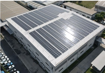
Example of renewable energy use (solar power generation system at our plant in Thailand)
